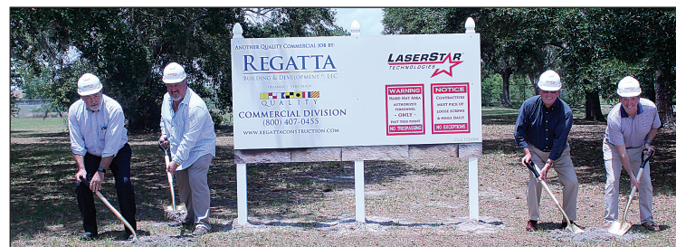
Groundbreaking at the Orlando facility expansion. The state-of-the-art facility will be completed later this year.
